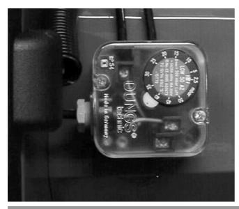
The air pressure switch is a differential pressure switch and monitors pressure at the forced-air burner.
